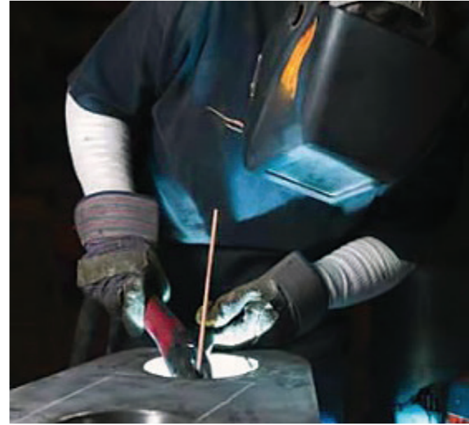
Bore repair / bushing replacement
