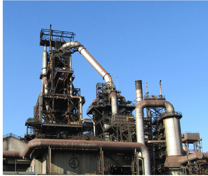
Tri-Ax Cyclone and modified downcomer
