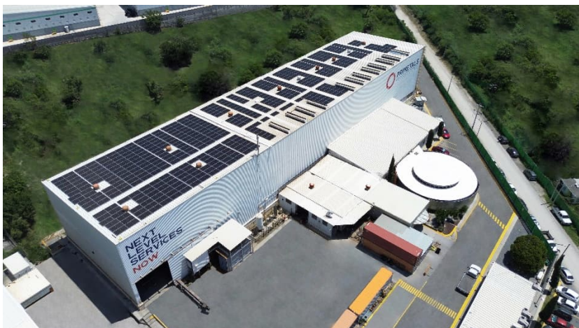
Primetals Technologies’ workshop in Apodaca, Nuevo Leon, Mexico.
