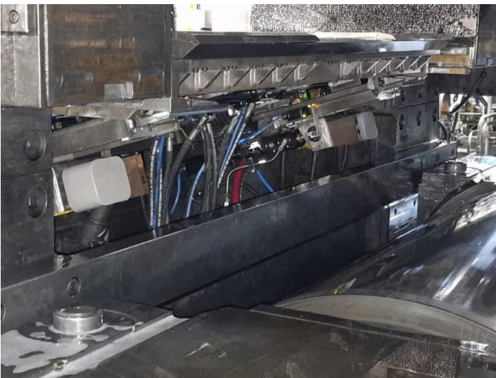
Inductor system from Primetals Technologies in operation at a customer's site.
