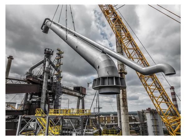
Construction of the gas cleaning plant from Primetals Technologies – a 1000-ton crane lifting the final piece of the downcomer into position.
