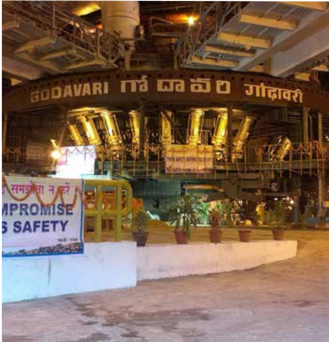
RINL Vizag Blast Furnace No.1 blow-in
