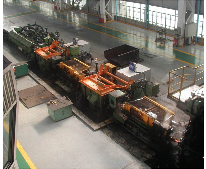
Morgan Vee pre-finishing mills
