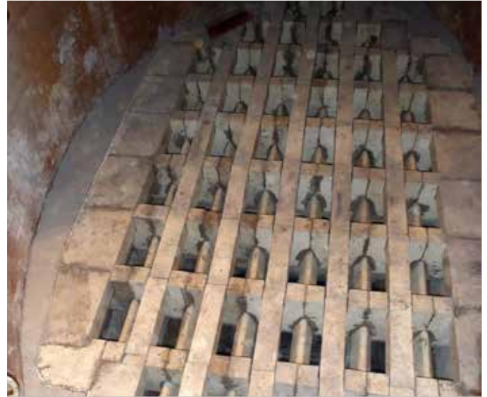
Repaired internal stove
