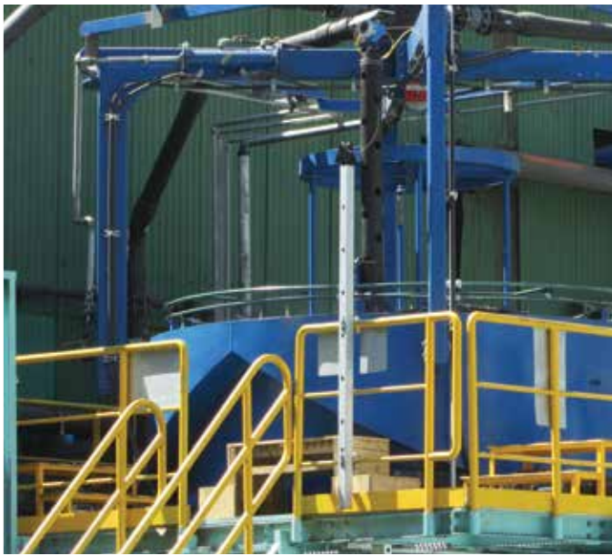
Hybrid Flotation cell installation
