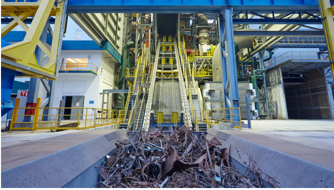
Automated scrap charging system via elevator
