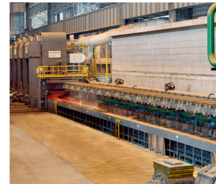
Laminar cooling section
