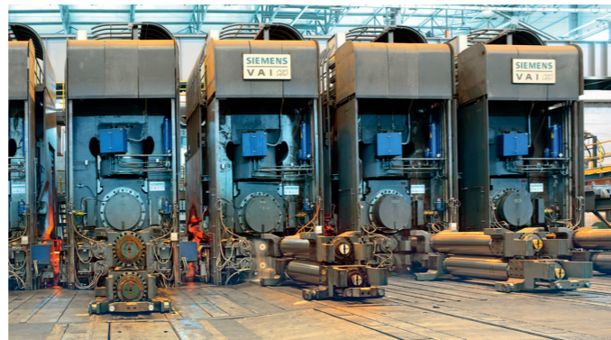
5-stand finishing mill
