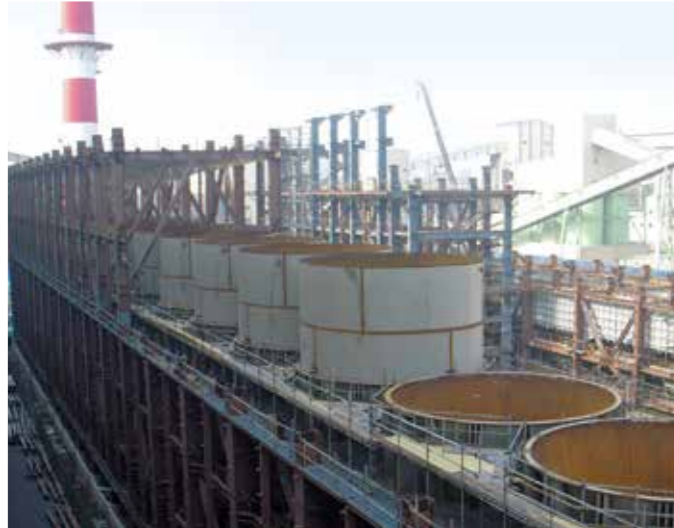
Proportioning bins under construction
