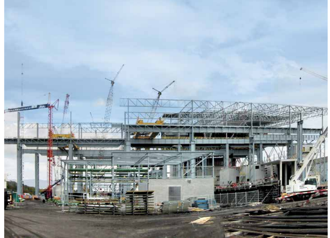
Installation of steel structure
