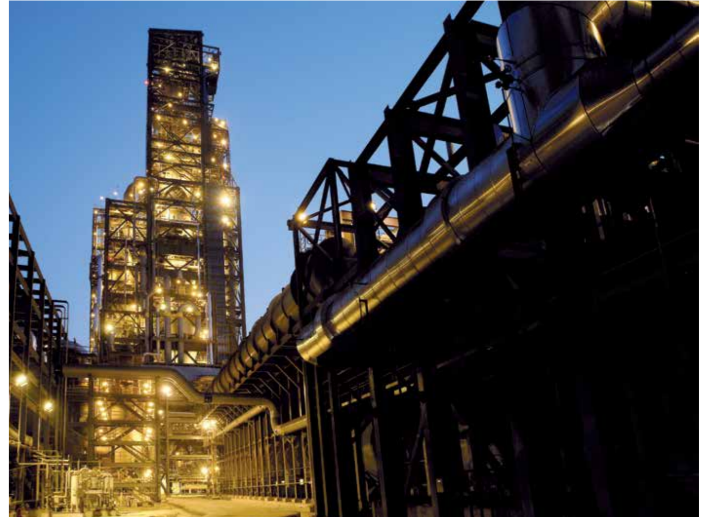
Bay steel structure, rolling mill
