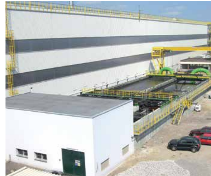
Water treatment plant for hot-strip mill (executed)
