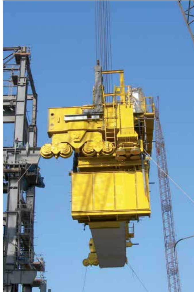
Lifting of crane bridge
