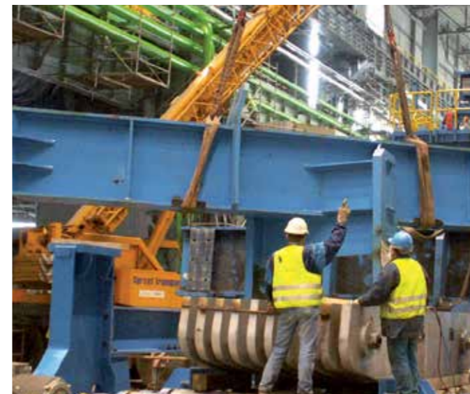
Installation of rolling mill
