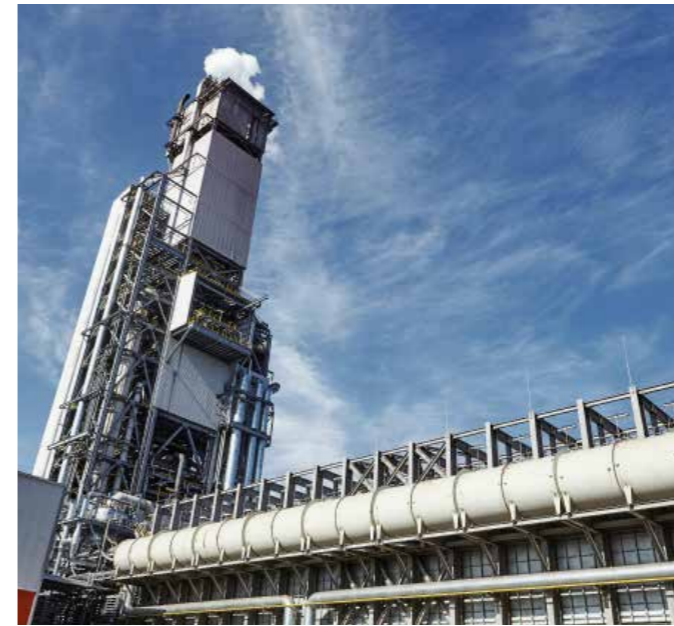
LGOK III MIDREX HBI PLant
