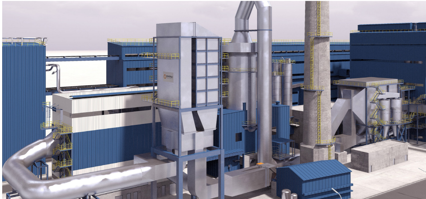
3D Modell of SCR DeNO x plant for sinter waste gas cleaning
