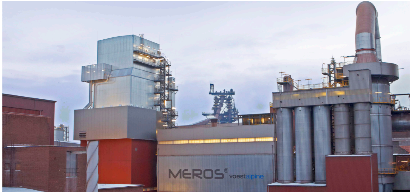
MEROS® plant at voestalpine in Linz, Austria
