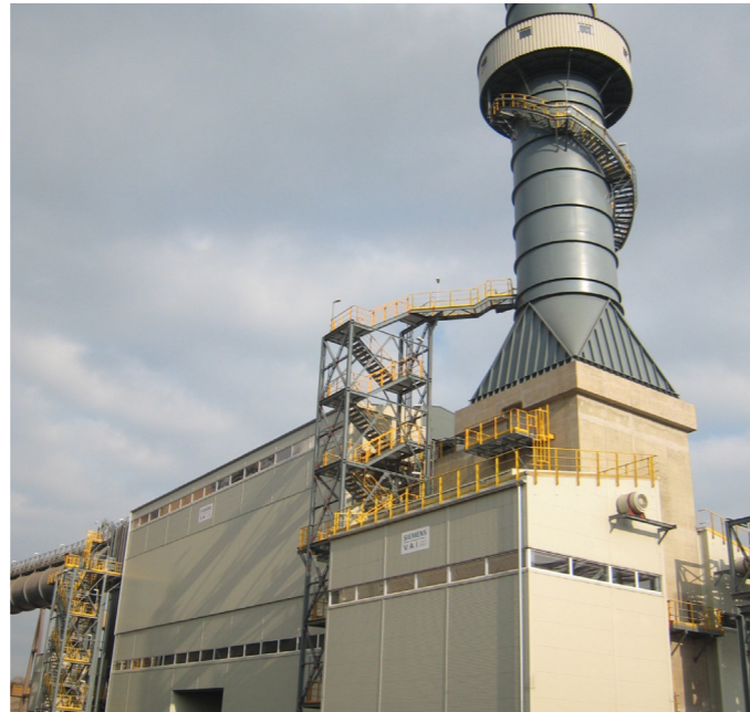
Fan house and stack
