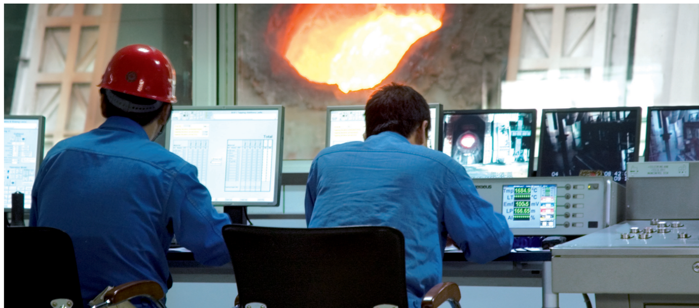
Converter control room at Taiyuan ISCO, China
