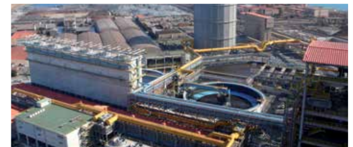
Water treatment, Posco, Pohang, South Korea
